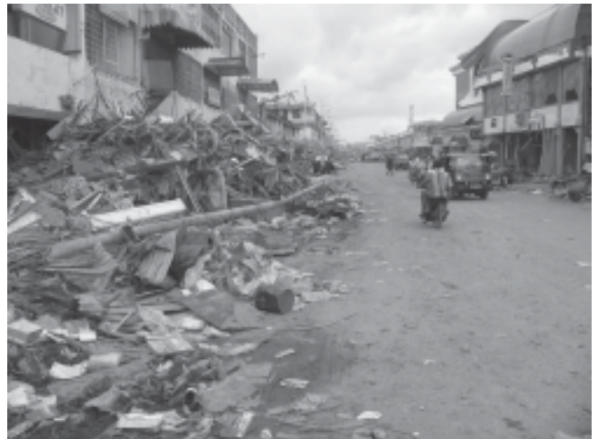
Fig. 3. The roads were slowly cleared to allow access by vehicles.
