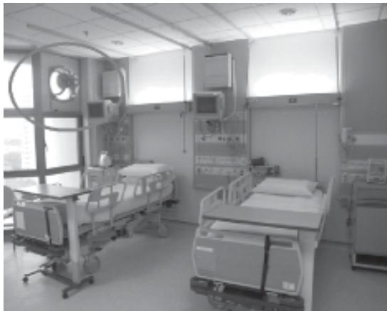
Fig. 2. An industrial exhaust fan (circle) was installed at the window to create negative pressure in the converted SARS cohort ICU.
