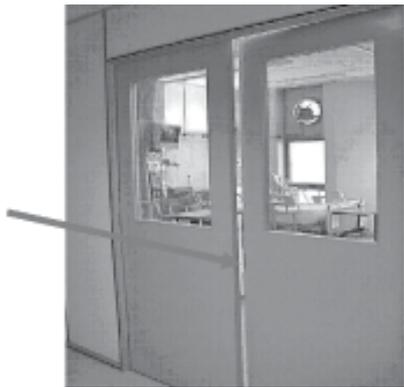
Fig. 1. Conversion of the 6-bed high-dependency room into a SARS cohort ICU room. Note the creation of a temporary partition, consisting of swing door with viewing glass window, at the original open entrance. The door remains slightly ajar (arrow) when there is negative pressurisation of the patients’ room.
